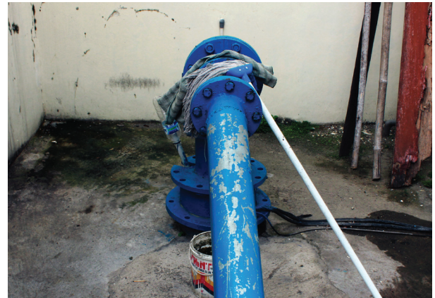
A deepwater well in the Mojosongo Kelurahan (neighborhood), such wells pump water from depths of 100-200 meters underground
