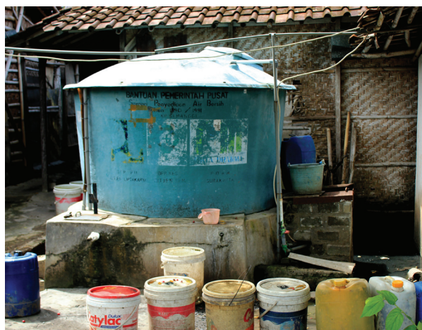
Public water hydrant at RW7, RT 3, Semanggi. Households fill containers and jerry cans for domestic consumption.
